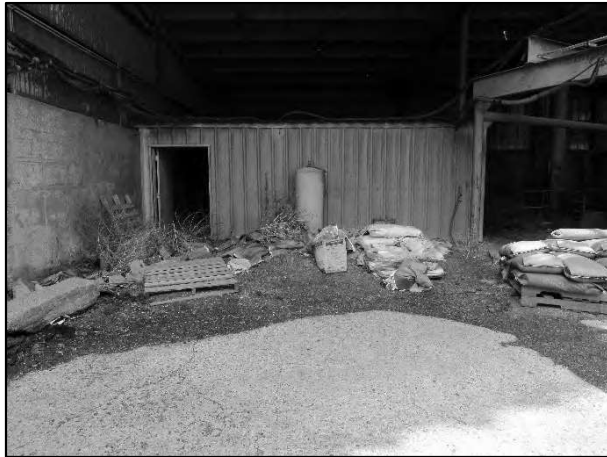
7M – Feed Mill – No Contributory Value
