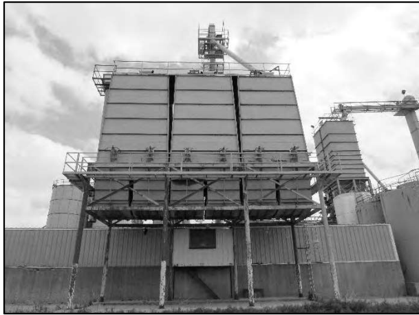
7M – Truck Load Out – No Contributory Value
