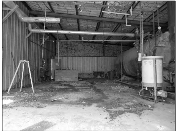
7M – Holman Boiler Removed – No Value
