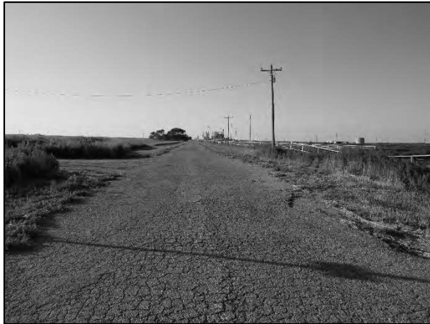
7M Feedyard – CR 15 Frontage Looking North
