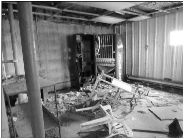
7M – Feed Mill – No Contributory Value
