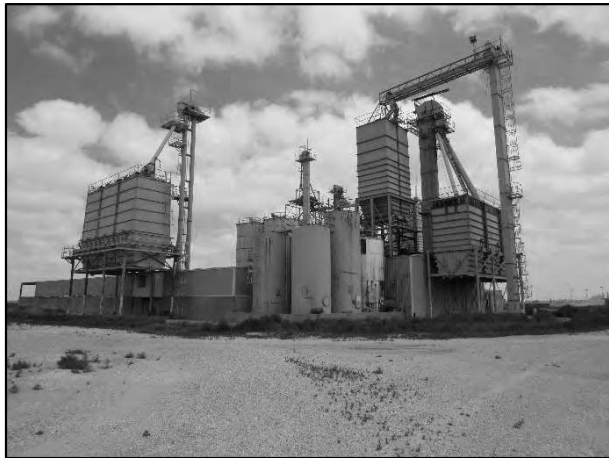
7M – Feed Mill – No Contributory Value
