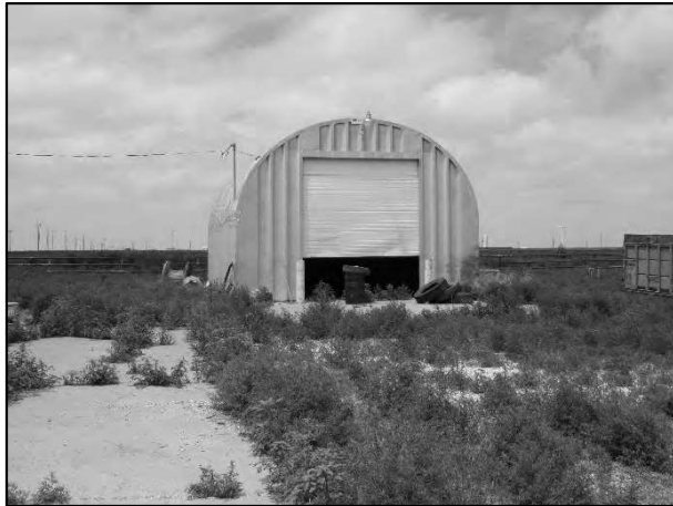
7M – Quonset - Contributory Value
