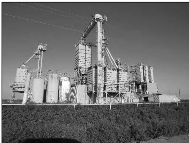
7M – Feed Mill – No Contributory Value
