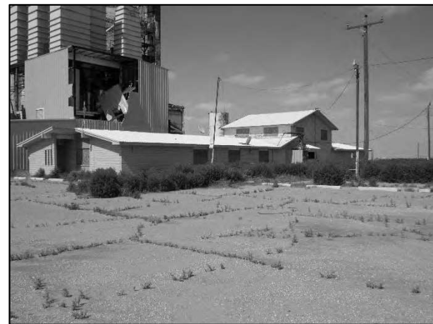
7M – Feed Mill/Office – No Contributory Value
