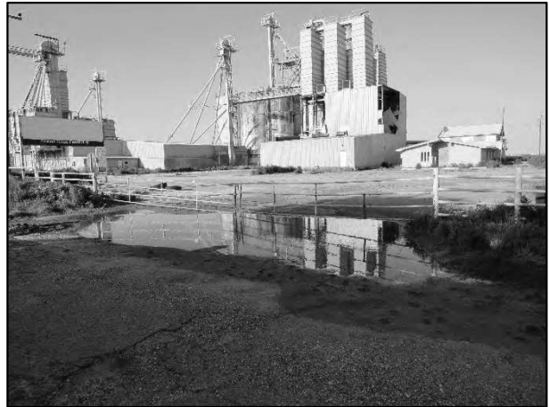
7M Cattle Feeders – Main Entrance Along CR 15
