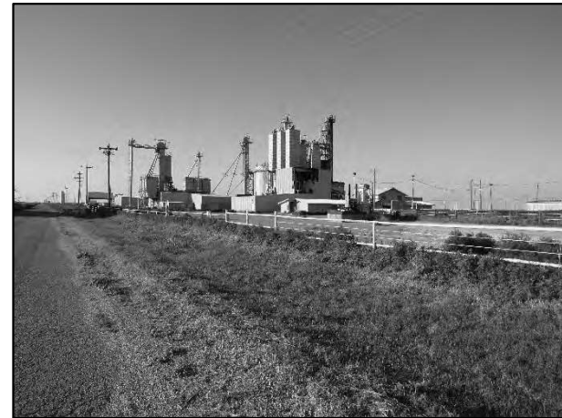
7M Feedyard – CR 15 Frontage Looking North
