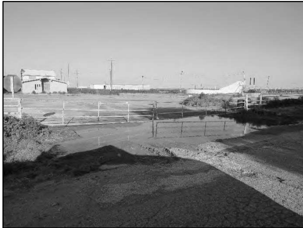
7M Cattle Feeders – Main Entrance Along CR 15
