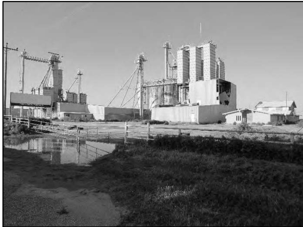
7M – Feed Mill – No Contributory Value
