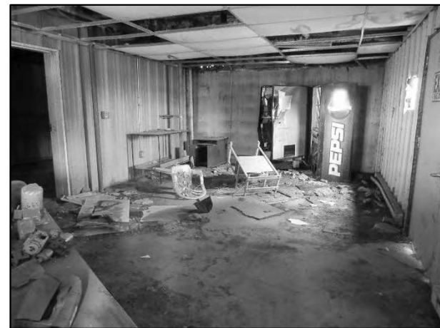
7M – Feed Mill – No Contributory Value
