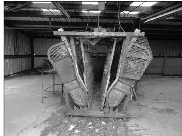
7M – North Processing Barn - Contributory Value
