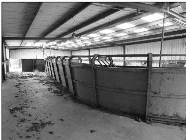
7M – North Processing Barn - Contributory Value
