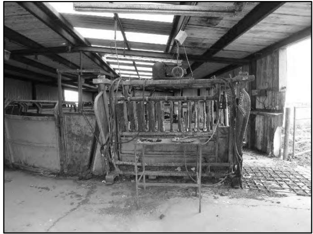
7M – North Processing Barn - Contributory Value
