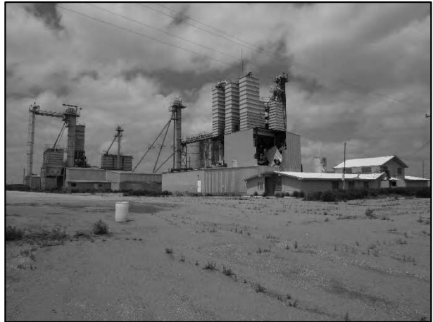
7M – Feed Mill – No Contributory Value
