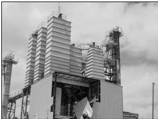
7M – Feed Mill Bldg./Ing. Bins/Legs – No Value
