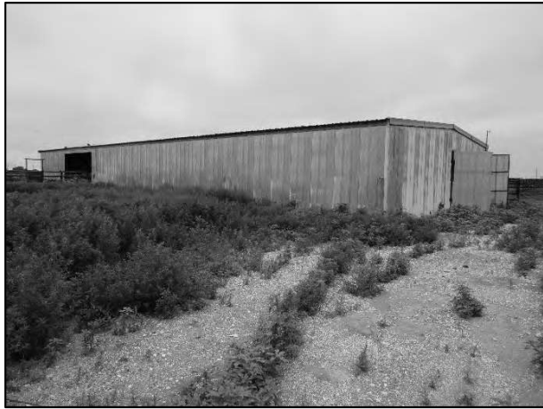
7M – North Processing Barn - Contributory Value
