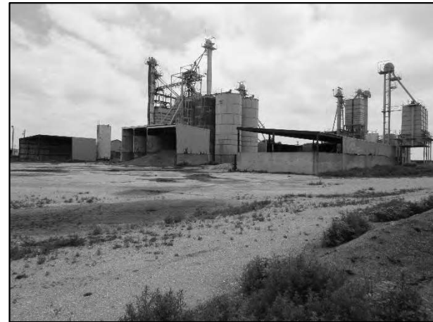
7M – Feed Mill – No Contributory Value
