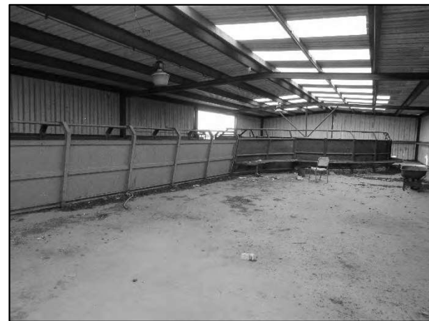
7M – North Processing Barn - Contributory Value
