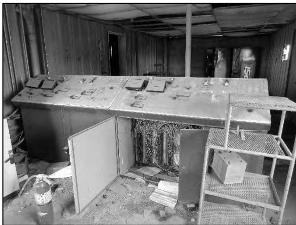
7M – Feed Mill – No Contributory Value
