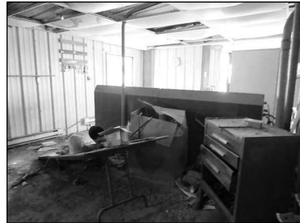
7M – Feed Mill – No Contributory Value
