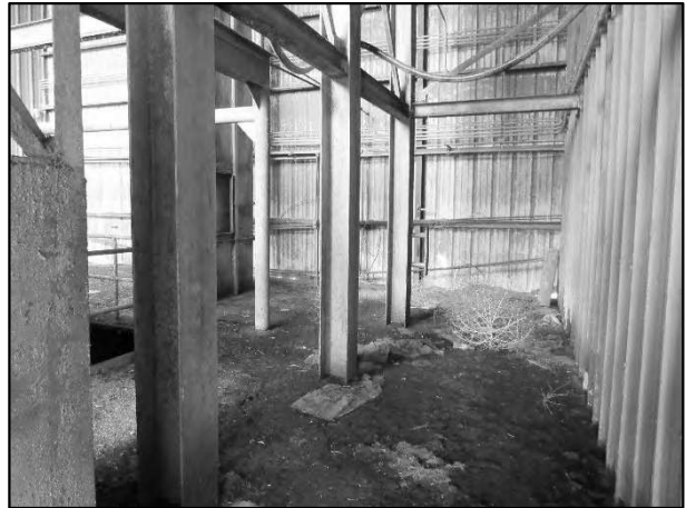
7M – Feed Mill – No Contributory Value
