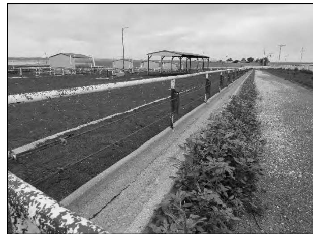
McClain Grow Yard – Concrete Feed Bunk / Pens
