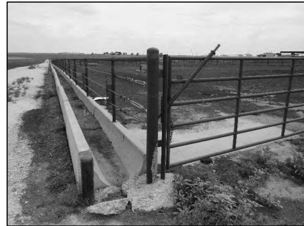
McClain Grow Yard – Concrete Feed Bunk / Pens
