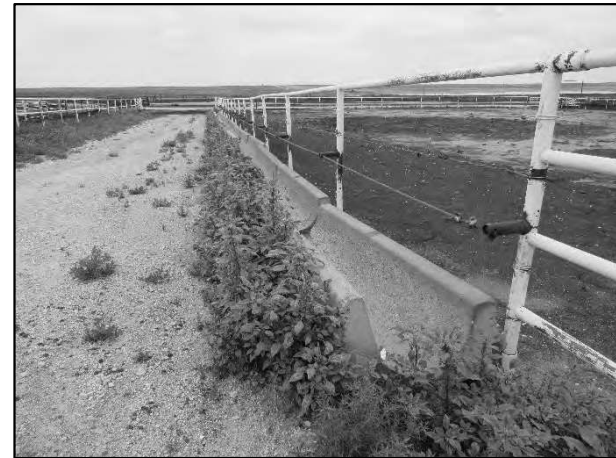
Def. Maintenance / Re-Level and Attach Bunk
