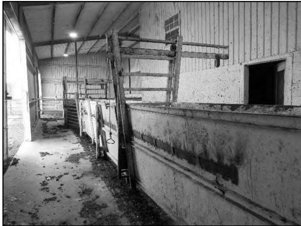
McClain Grow Yard – Processing/Hospital Barn
