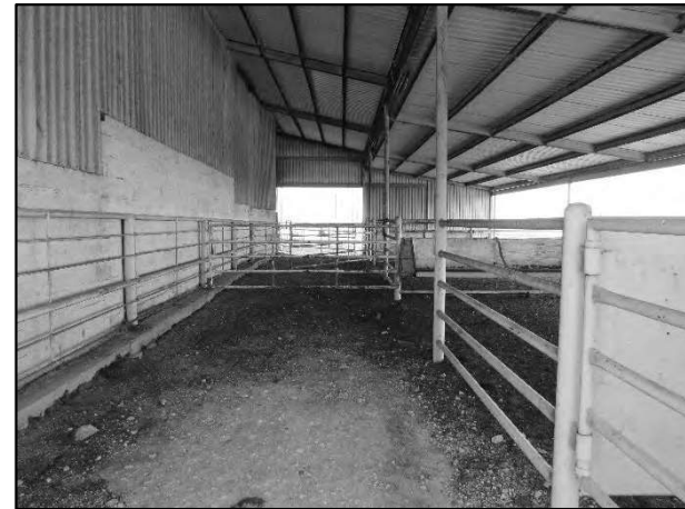
McClain Grow Yard – Processing/Hospital Barn
