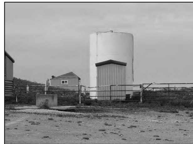
McClain Grow Yard – Water System
