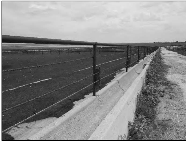
McClain Grow Yard – Concrete Feed Bunk / Pens
