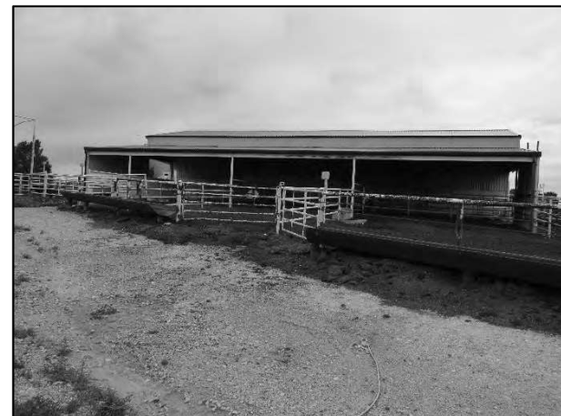
McClain Grow Yard – Processing/Hospital Barn
