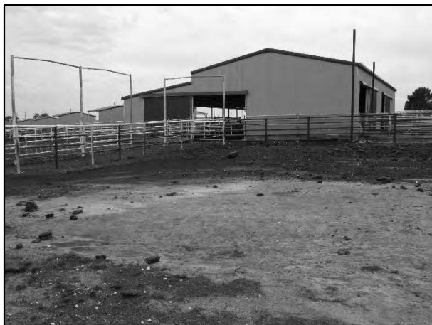
McClain Grow Yard – Processing/Hospital Barn
