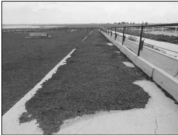
McClain Grow Yard – Concrete Feed Bunk / Pens
