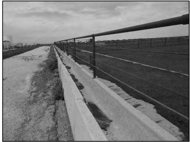
McClain Grow Yard – Concrete Feed Bunk / Pens
