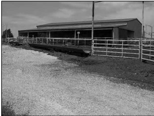
McClain Grow Yard – Processing/Hospital Barn
