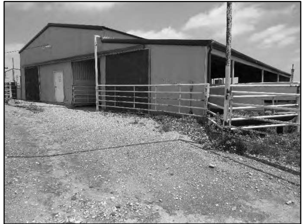
McClain Grow Yard – Processing/Hospital Barn
